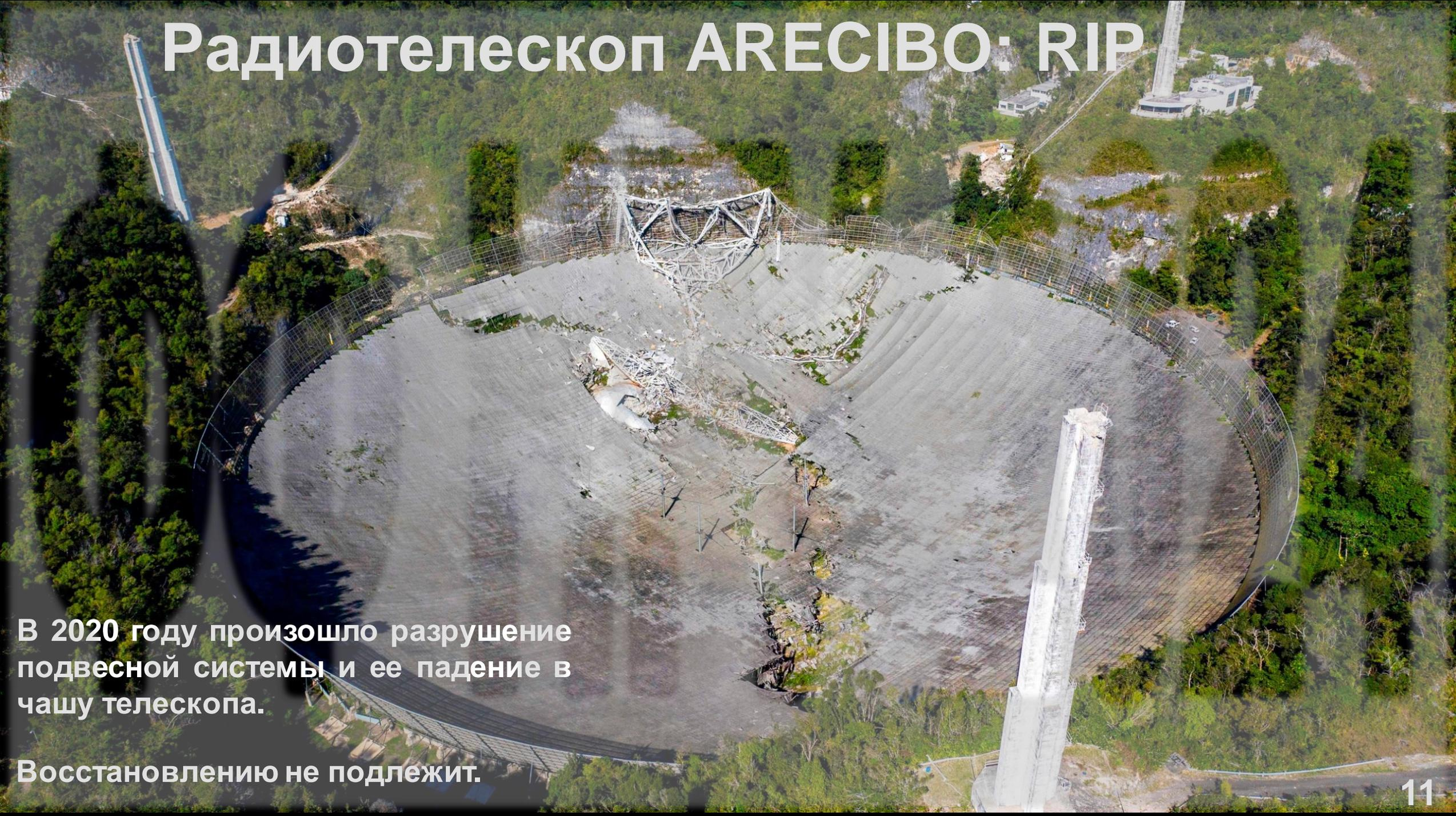
An aerial photograph of the Arecibo radio telescope dish, showing significant damage to the central suspension system and the surrounding structure. The dish is surrounded by dense green forest. In the background, there are some buildings and a tall tower.
